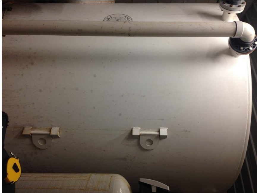
Figure 7: 300 gallon hot water storage tank
