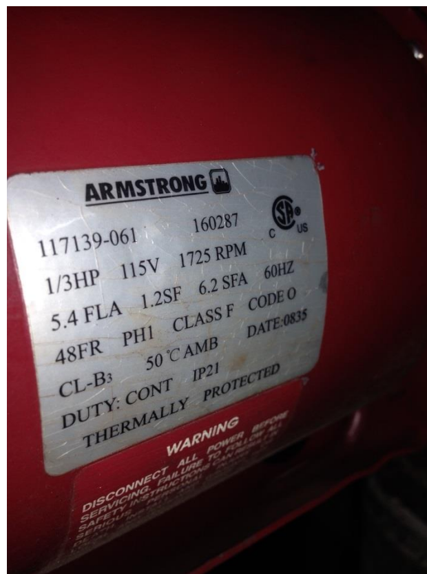
Figure 4: Marginal HP Pump Motor
