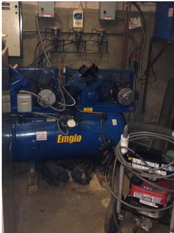
Figure 8: Pneumatic air compressor
