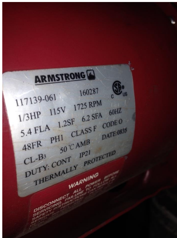
Figure 4: Marginal HP Pump Motor
