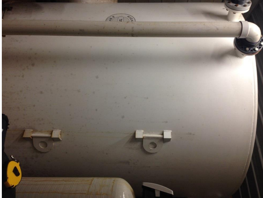
Figure 7: 300 gallon hot water storage tank
