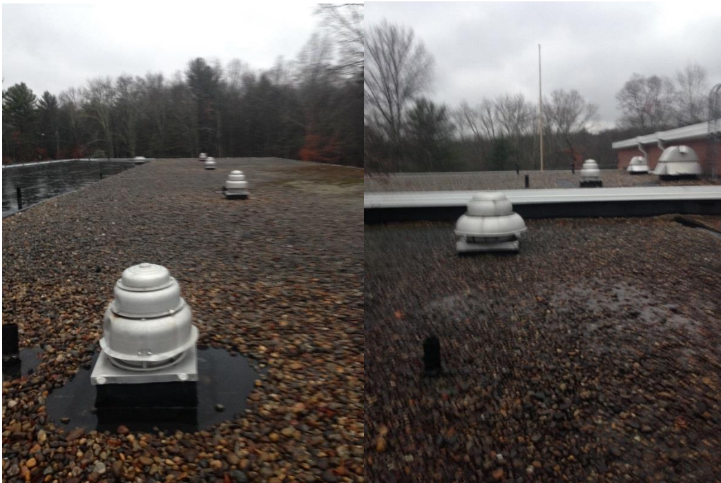
Figure 6: Exhaust hoods on roof
